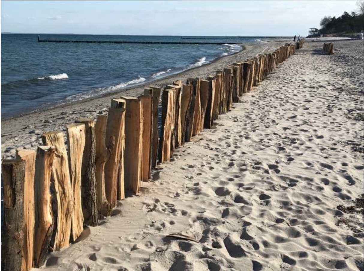
Abb. 15: Palisaden Kellenhusen (Foto: G. Heerten, maritime.geotechnical.consulting)
